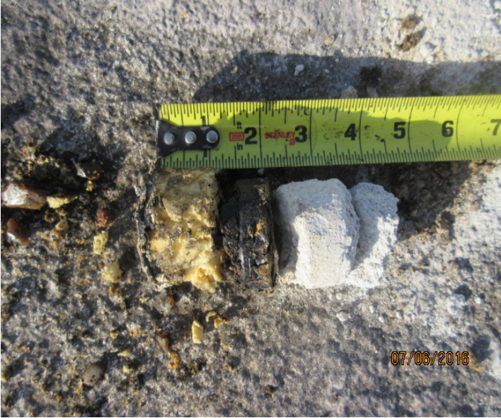
3. ROOF CORE ON AREA "D"
