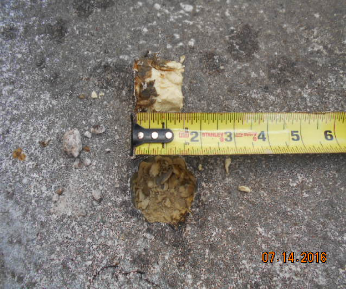
4. ROOF CORE ON AREA "H"
